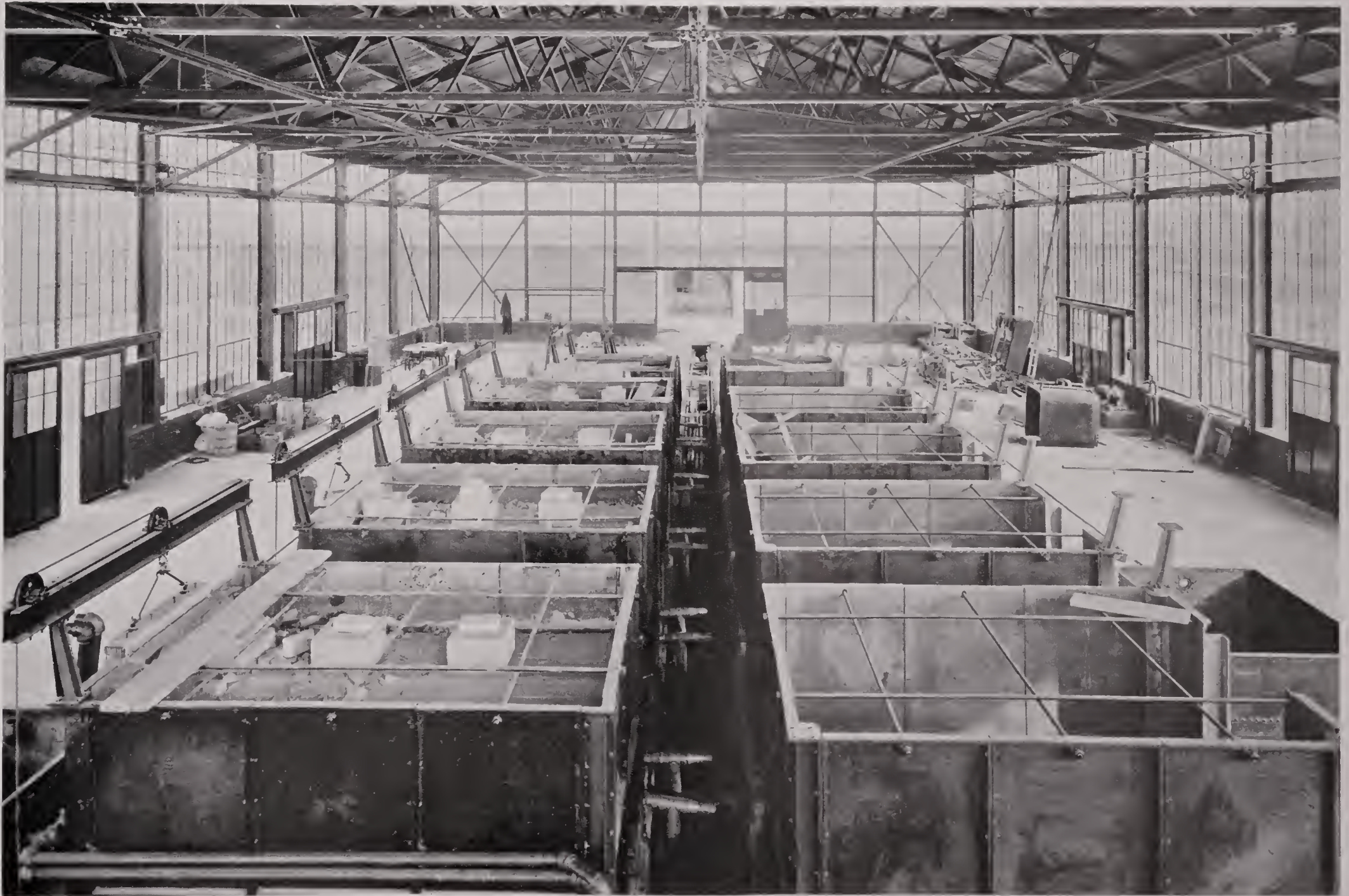
INTERIOR OF THE HEAT TREATING PLANT
